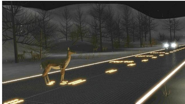
Figure 4: Warning appears on road to alert driver
