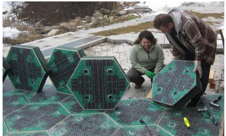
Figure 2: The Brusaw's installing solar road panels in a driveway
