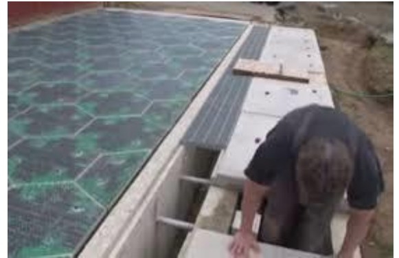
Figure 5: Mr. Brusaw working on a cable corridor
